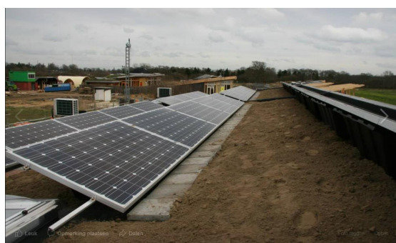
Rooftop solar-modules during installation
