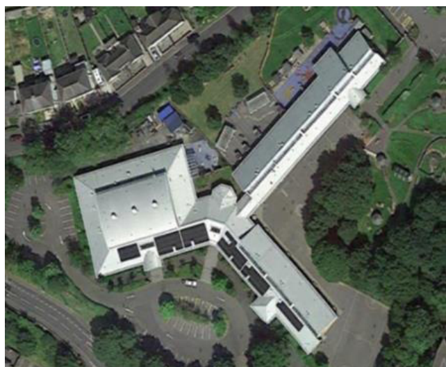
Aerial view of Ysgol y Bedol PV E.CO
